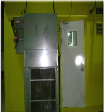
Air Cooled Package Unit
