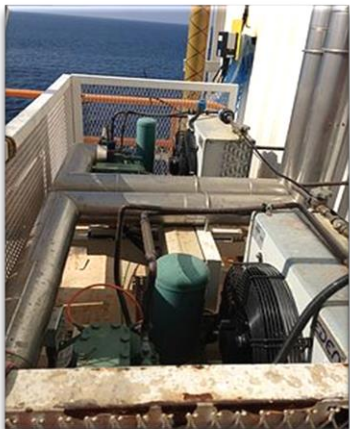
Air Cooled Condensing Unit
