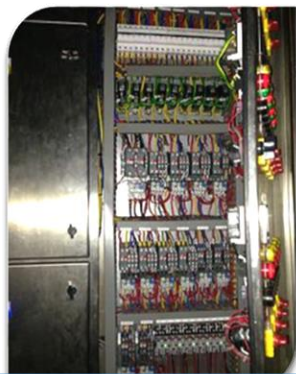
MCC Starter Panel
