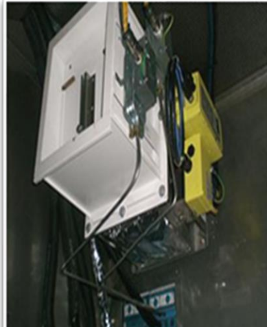
Pressurization Damper & Flow Switch
