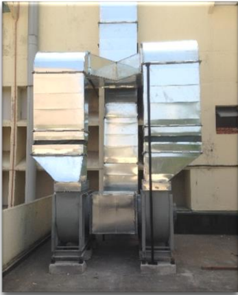
Ventilation Ducting
