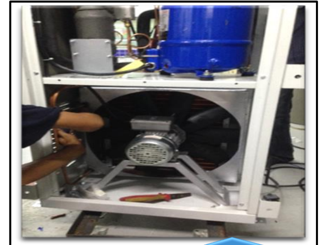
PSR MELAKA - CRANE AC UNIT FAN INSTALLATION
