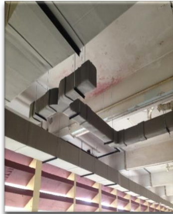
Insulated Ducting
