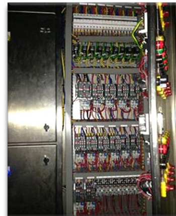
SS316L MCC Starter Panel
