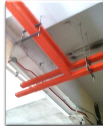
Power Cable Trunking
