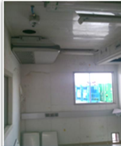
Air Cond Unit
