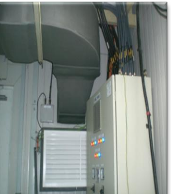
Ducting & Cable Glanding
