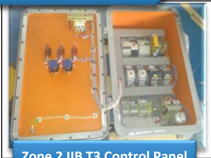
Zone 2 IIB T3 Control Panel
