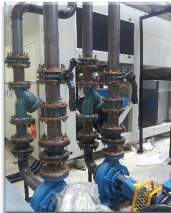
Chiller Water Piping
