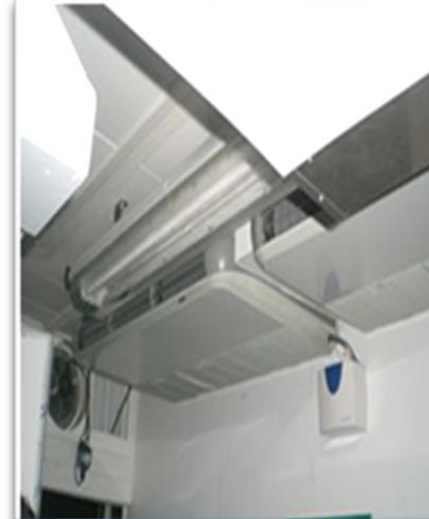
Air Cond Unit & Drain Pump
